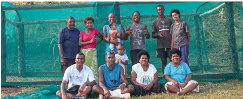
Figure 9: Construction of Solevu Yaubula Nursery at Cavaga Village (Bua Province)
