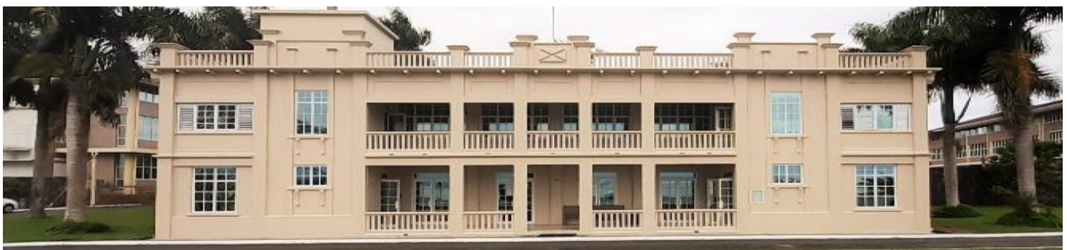
Figure 21: Veivueti Building (TTFB)
